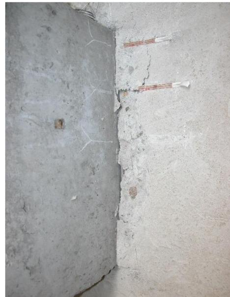
b) column cracks and spalls
